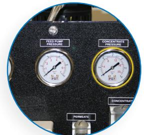
Liquid Filled Panel Mounted Concentrate Pressure Gauge
